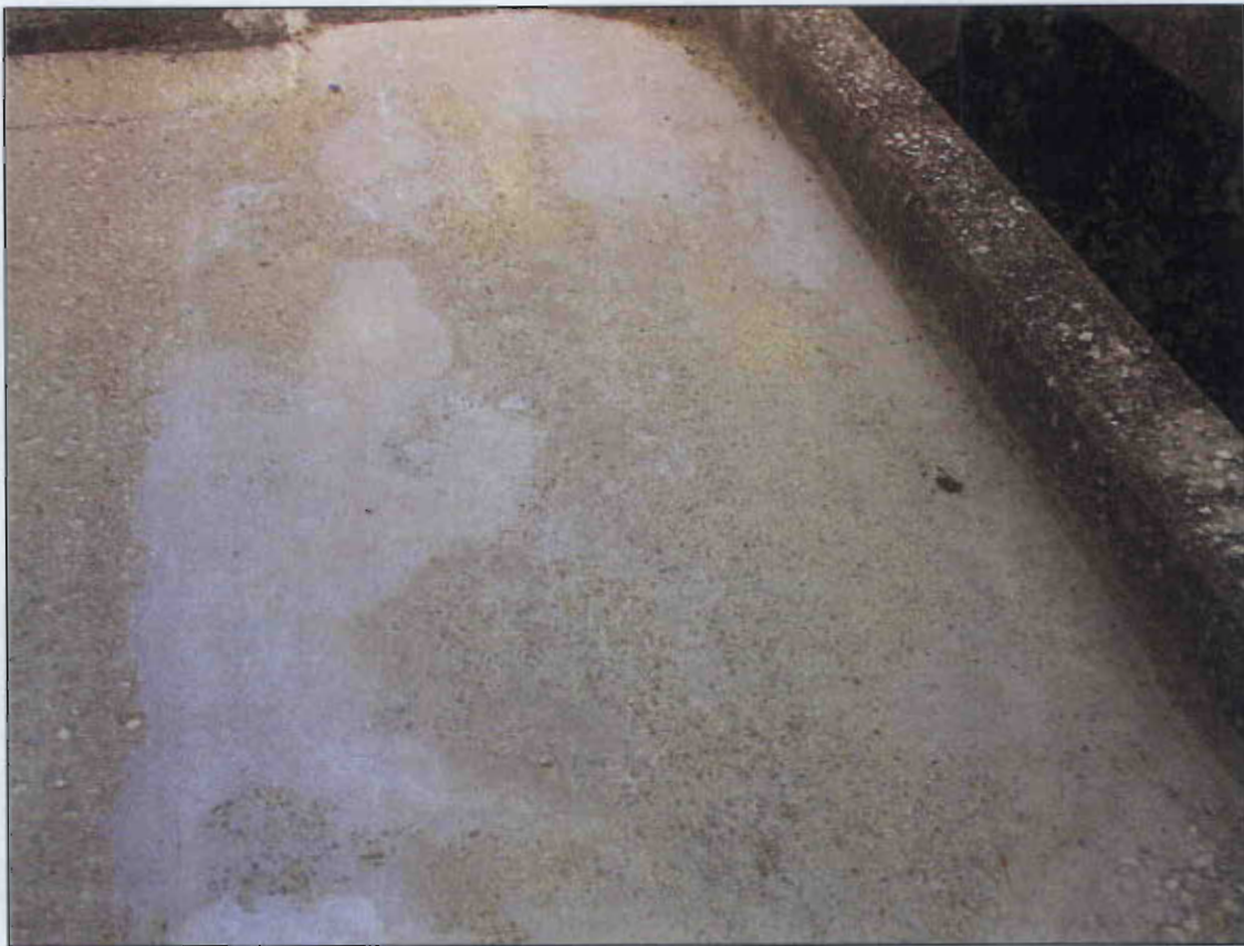
PATCH IN THE RIGHT SIDE OF SPAN 2 AT END BENT 2
