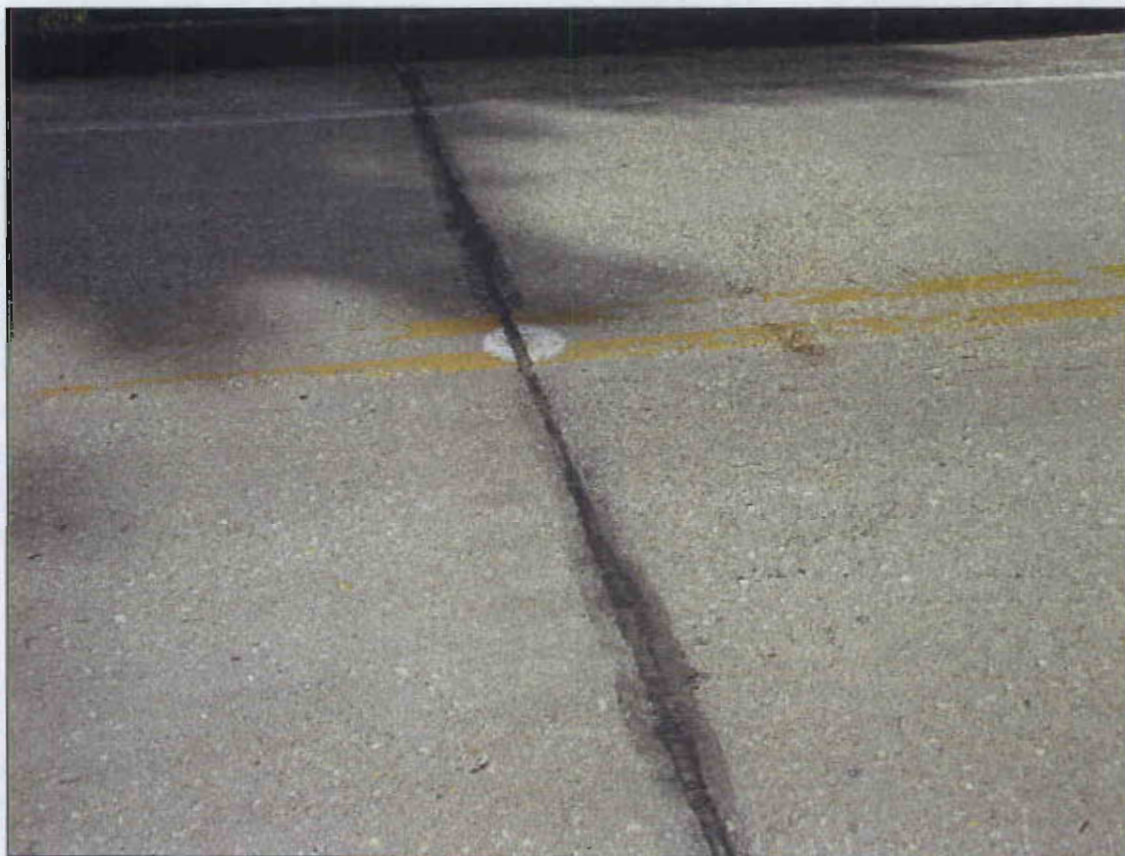
JOINT AT INTERIOR BENT
