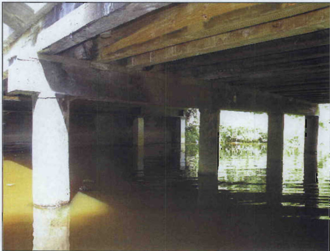
INTERIOR BENT SPAN 2 SIDE
