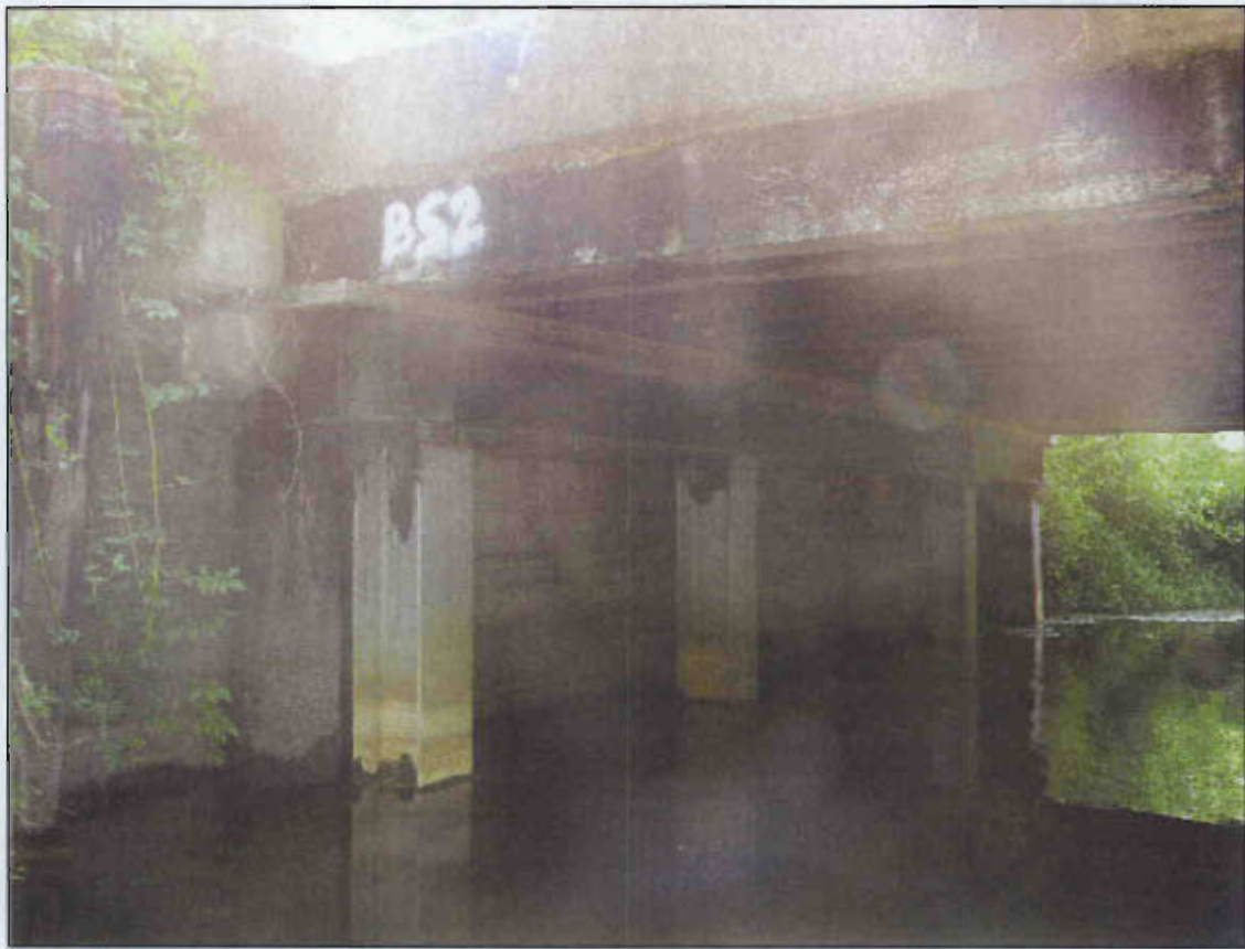
END BENT 2 OVERVIEW
