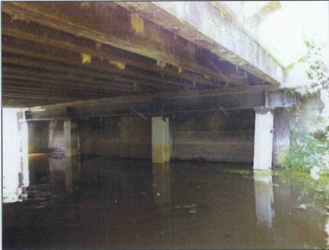
END BENT 1 OVERVIEW
