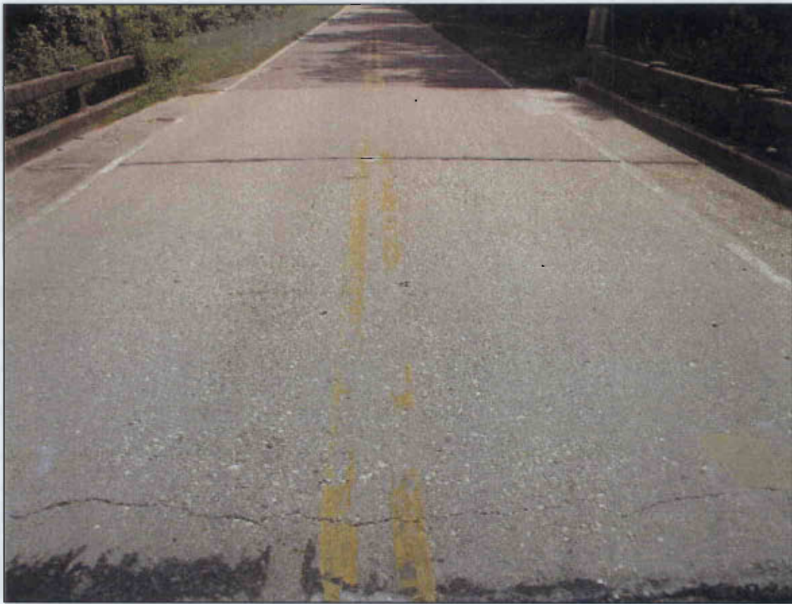
TOP OF DECK OVERVIEW
