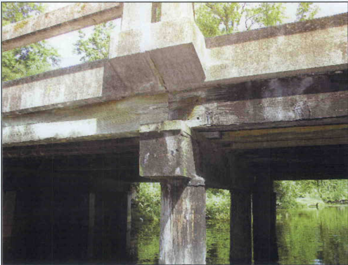
SUPERSTRUCTURE OVER END OF CAP
